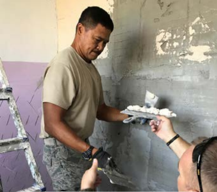
U.S. Air Force Tech. Sgt. Raymond Gipaya, a Structural Specialist, with the 144th Civil Engineer Squadron trues a soviet era wall prior to tiling at a school near Chisinau, Moldova. (US Air National Guard photo by Master Sgt. David J. Loeffler)
